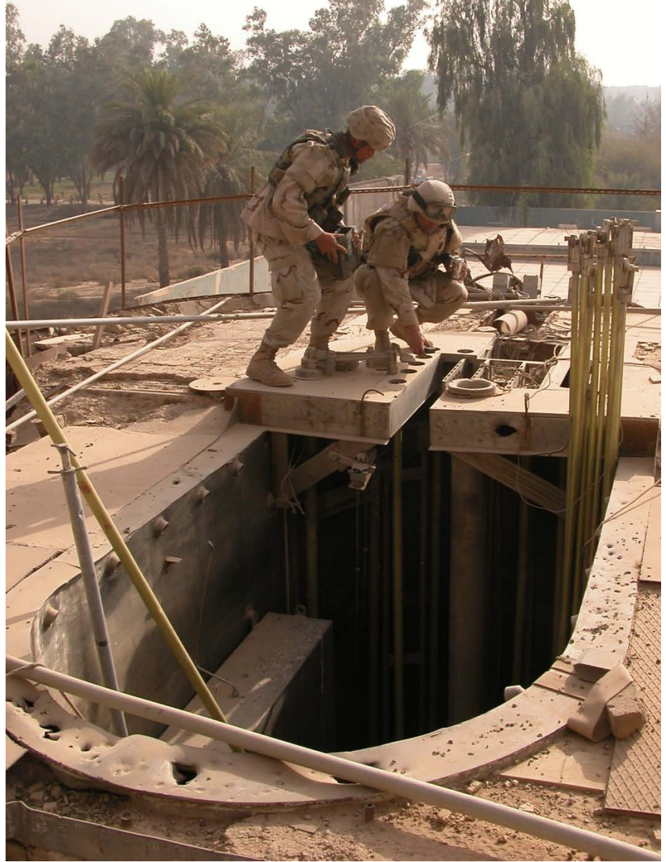
Atop the cooling tower (IRT 5000)
